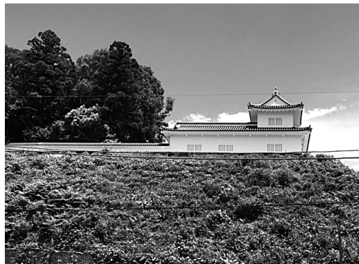
Two-story corner tower (rebuilt)
